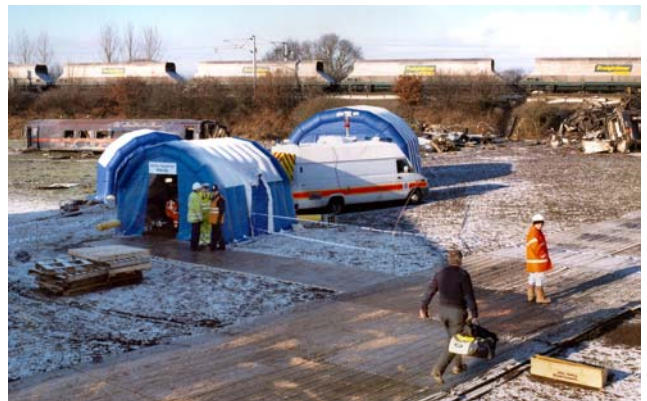
Airesshelta inflatable buildings in action at the scene of the Selby rail crash
